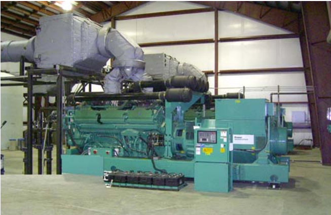
Cummins QSK60-G6 diesel engine with CRT filter converter (top). Urea injector, electronic controls (not shown) and SCR catalytic converter (bottom).
