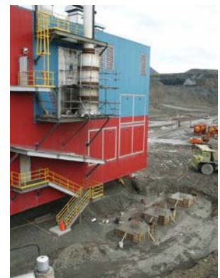
Installation of the power house
