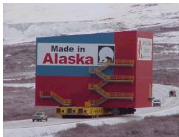
Power house enroute to the site
