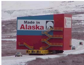
Power house enroute to the site
