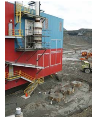
Installation of the power house
